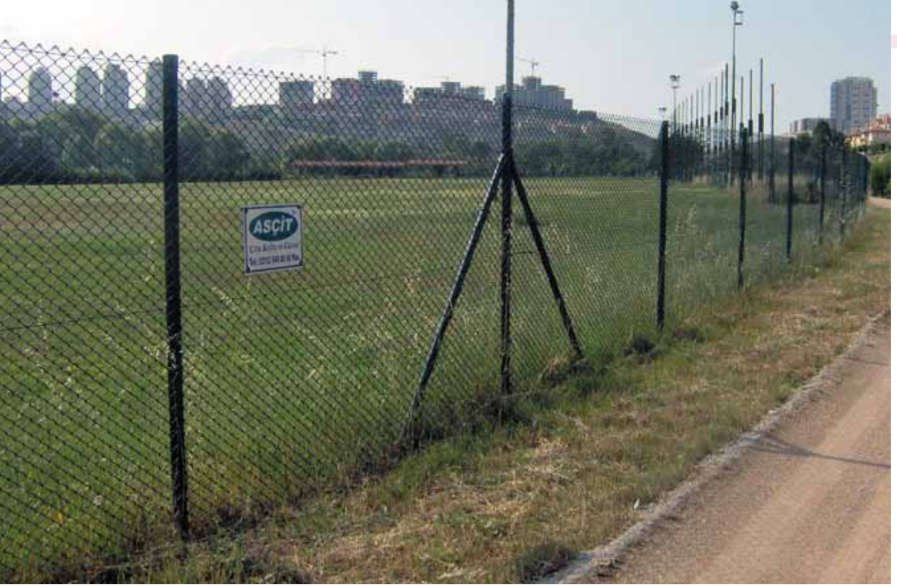
Galvaniz üzeri PVC kaplı örgü tel uygulaması, polyester kaplı direk ve payandalar. Galvanized and PVC coated chainlink fence application - polyester coated post & braces.
